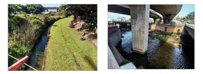
Figure 2.12 Degradation of the lower Baakens. L: The canalised estuarine section to the west of the Tramways building. R: The estuary below the freeway (low tide).
