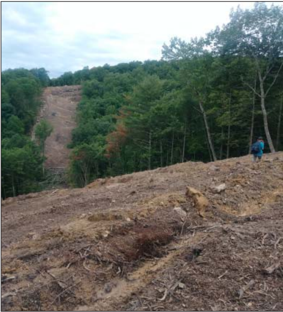
125 ft. wide right-of-way for the Atlantic Coast Pipeline
