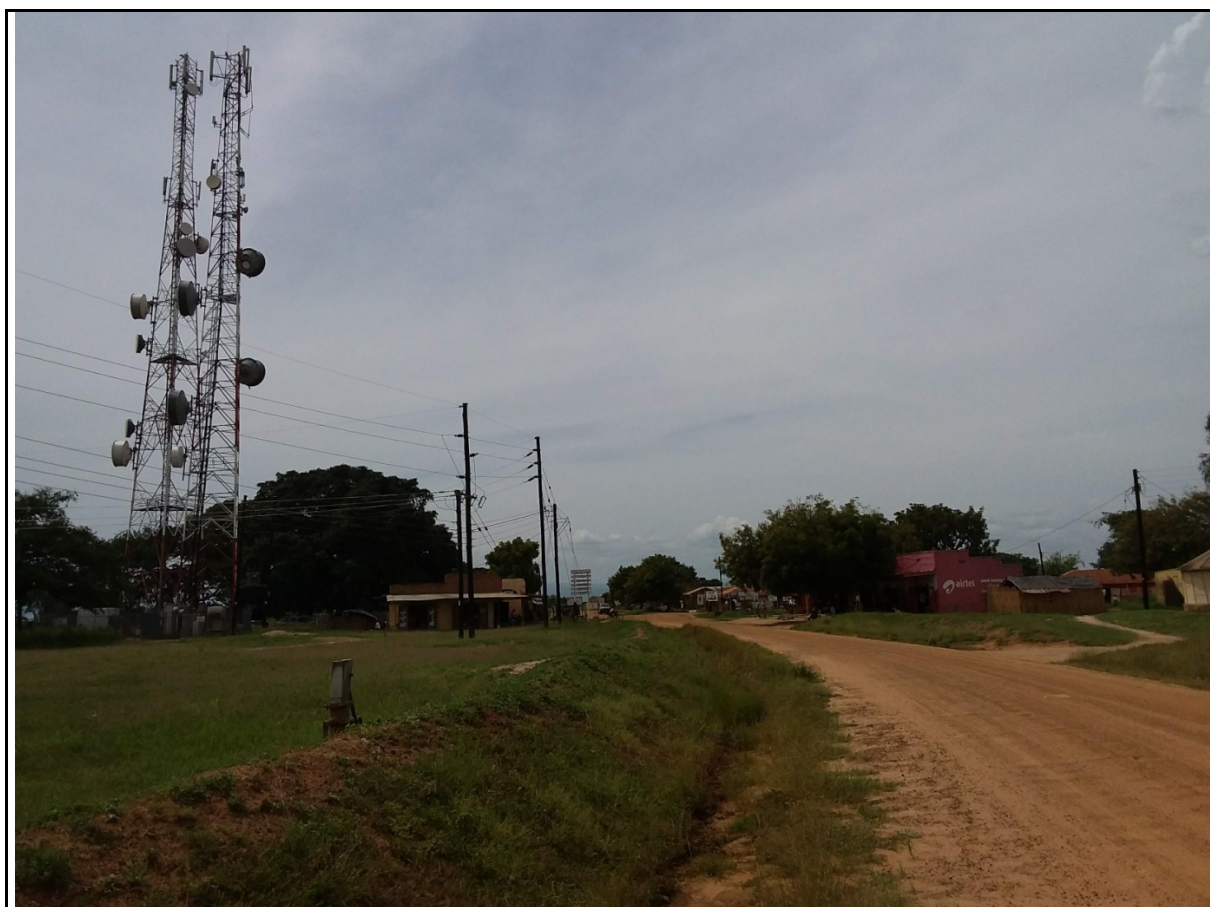
Figure 6.4-23 Power Cables in Buliisa, Buliisa District (KP8)
