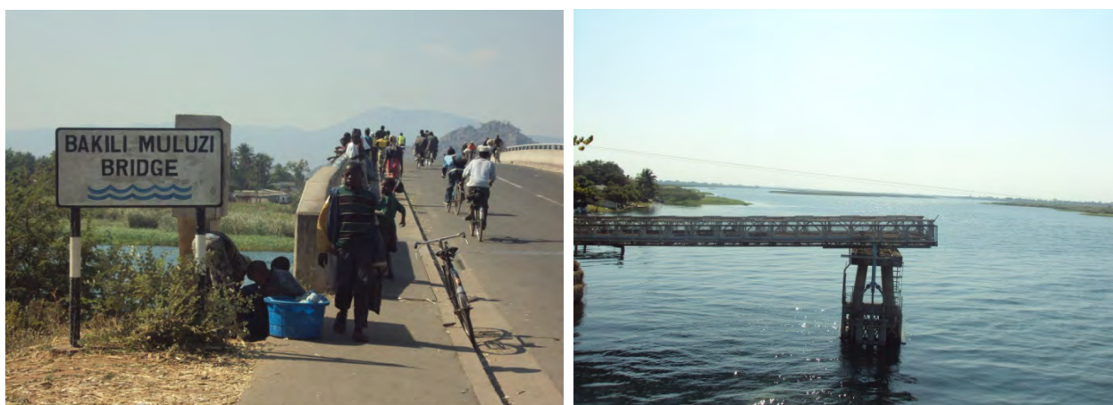
Figure 5. Bakili Muluzi Bridge (first and new bridge on the Shire River from mouth) – RIGHT: part of the old bridge (Photo: F. Kapute)
