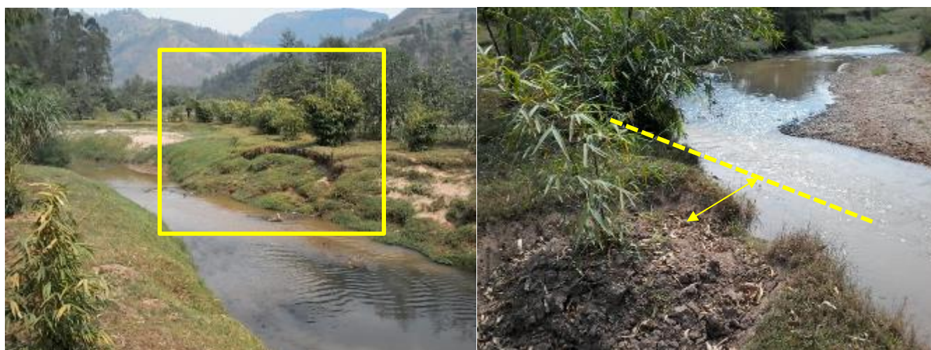
FIGURE 2-56 THE BAMBOO SEEMS TO BE EFFECTIVE FOR A LOCALISED AREA, AS INDICATED IN THE YELLOW BLOCK WHERE A BANK HAS SLUMPED UP UNTIL THE BAMBOO PLANT. THE YELLOW ARROW INDICATES THAT THE BANK HAS ERODED UP UNTIL THE BAMBOO PLANT (PICTURE: JULY 2017)
