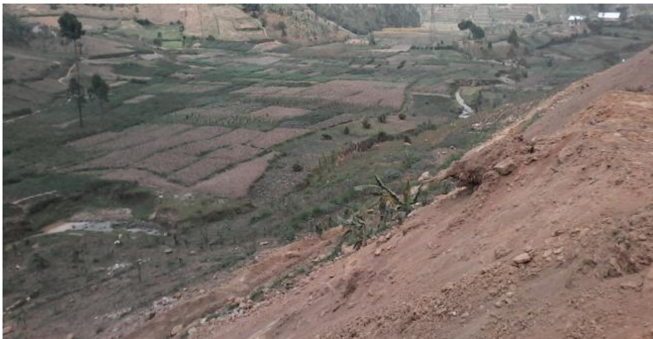
Figure 2-71: Cut material from road construction dumped on road side on a slope
