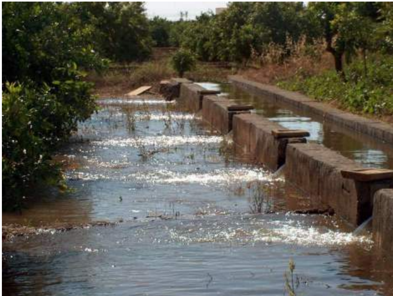
Figure 33. Riego “a manta” (flood irrigation). From the ditch to the field. Source: Real Acequia de Montcada.
