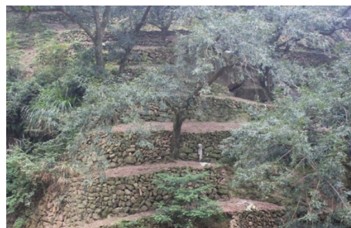
Figure 36. Manmade terraces to prevent the soil erosion
