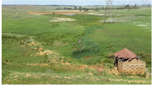
Smaller dam downstream of the upper dam.
