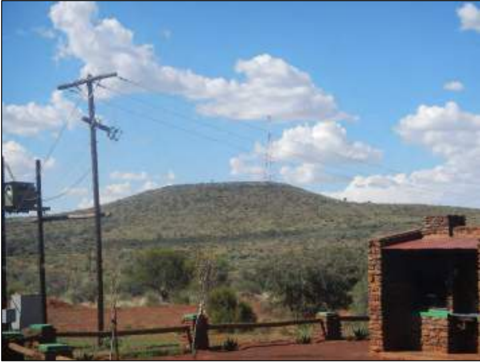
Figure 32: Typical view of some of the linear elements which are present at the Red Sands Country Lodge (SR2)
