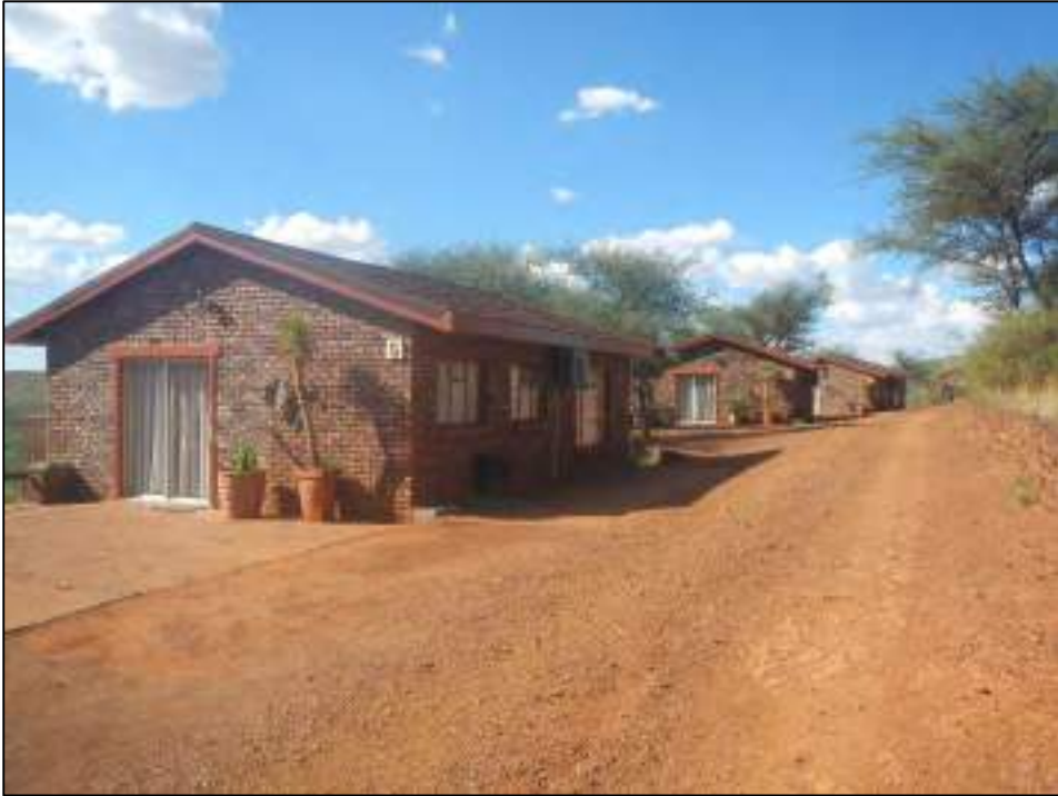
Figure 31: View of some of the chalets at the Red Sands Country Lodge (SR2)
