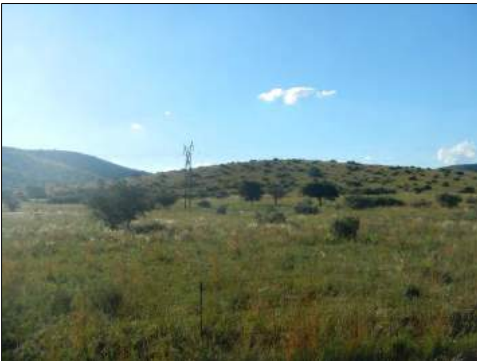
Figure 14: Typical view of the existing medium voltage power lines which can be found within parts of the study area
