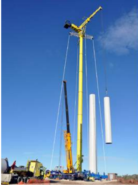
Figure 6: Cranes at work
