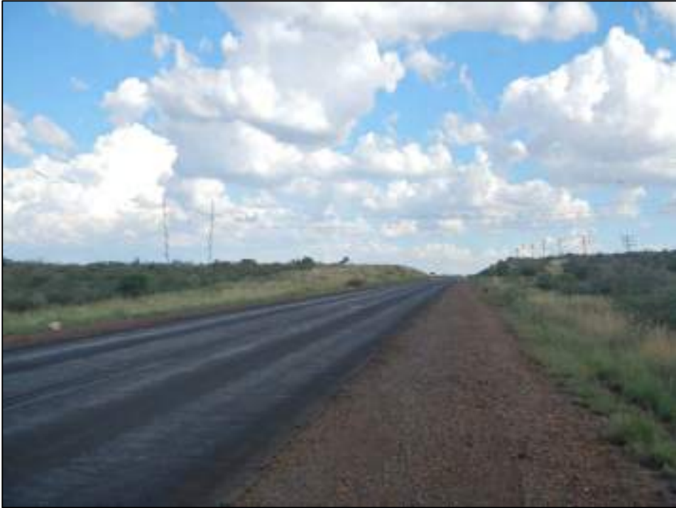
Figure 36: Typical view of the high voltage power line which is visible from sections of the N14 national route
