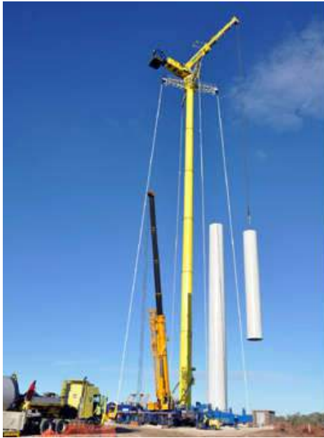
Figure 6: Cranes at work
