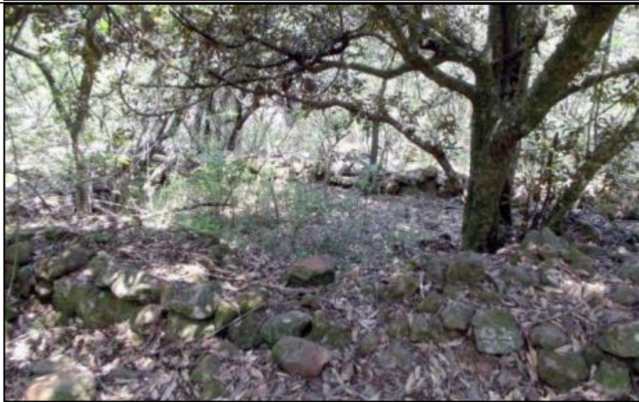
Photo 4.9.1 Photos of typical stonewall structures
