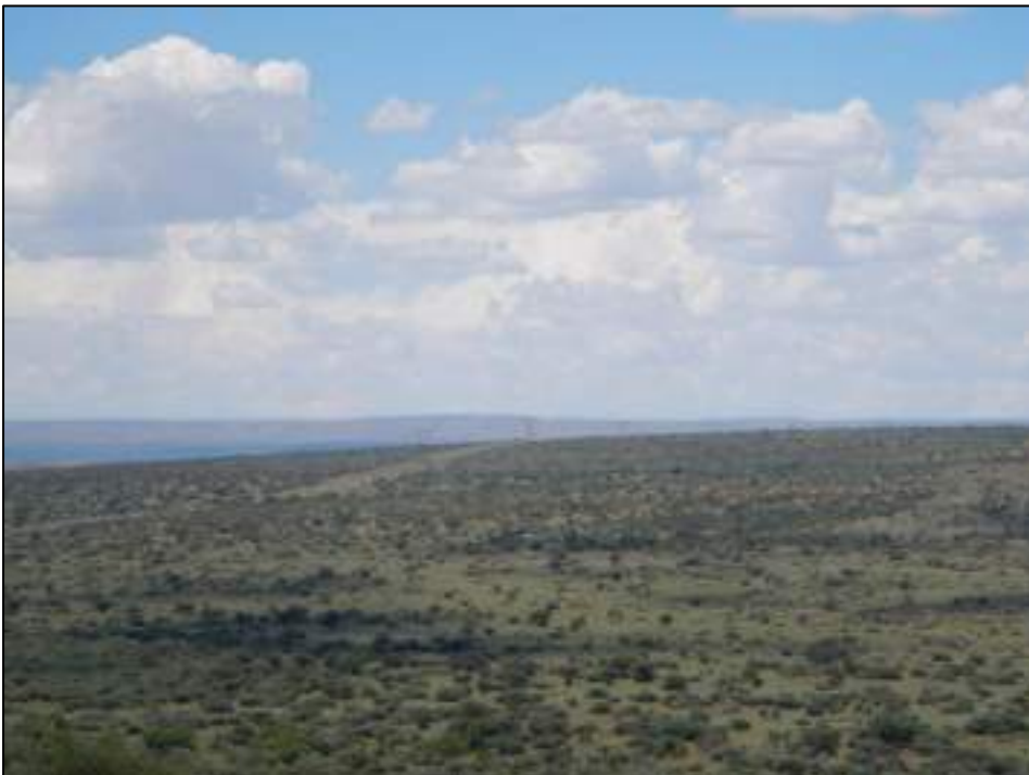
Figure 24: Typical view of the other high voltage transmission power lines which traverse the study area
