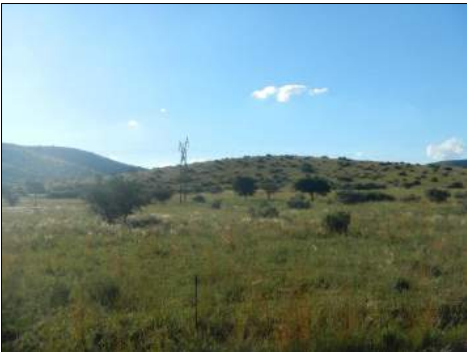
Figure 14: Typical view of the existing medium voltage power lines which can be found within parts of the study area
