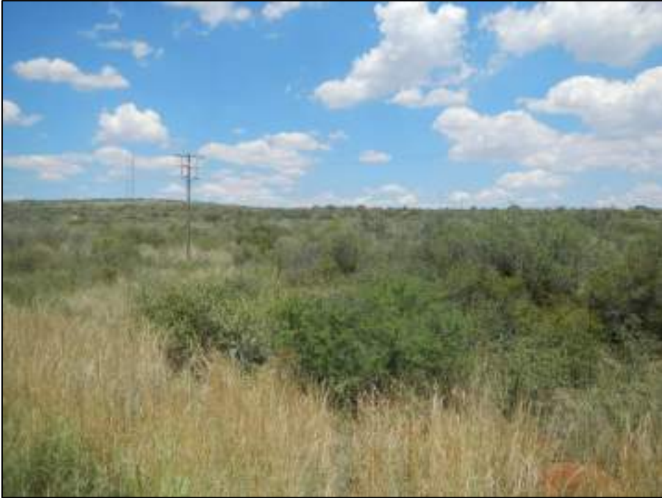
Figure 13: Typical view of the telephone lines which can be found within the study area
