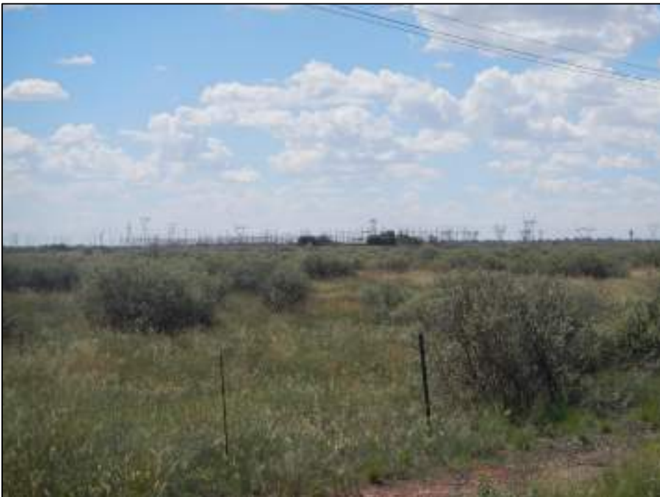
Figure 26: Typical view of the Ferrum Substation
