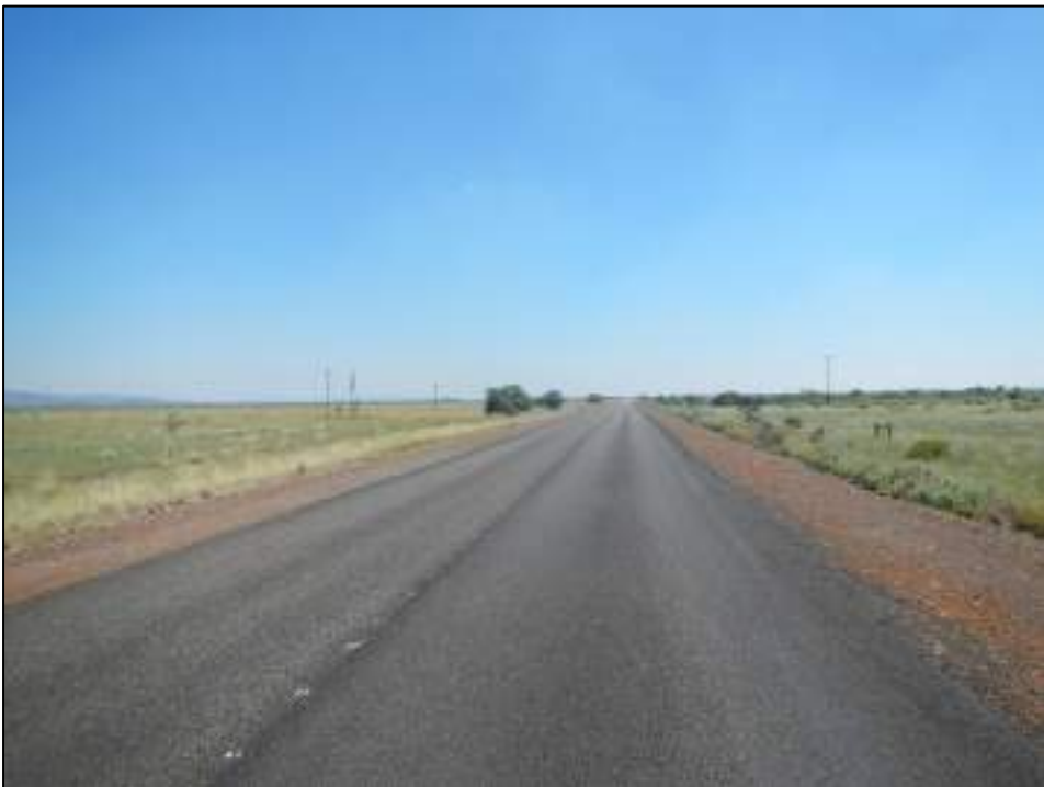
Figure 20: Typical view of the R31 main road
