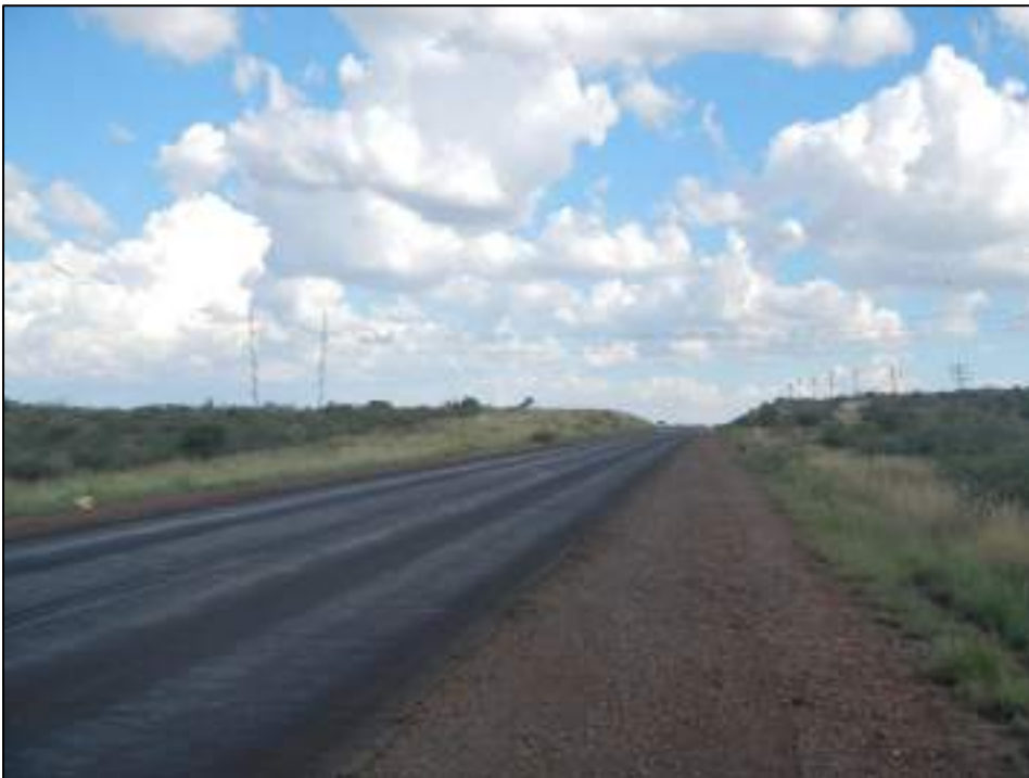
Figure 29: Typical view of a high voltage power line which is visible from sections of the N14 national route
