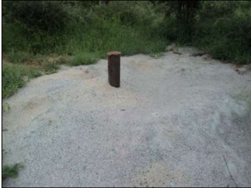
Fig. 15. Site SO 7. Photo of an existing borehole.
