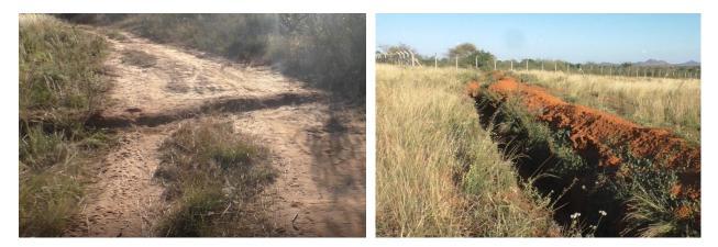
Figure 2: Road water harvesting intake and collection structures
