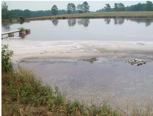
Figure 2. Swine waste lagoon that receives liquid part from the solid-liquid separator.
