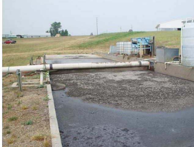
Figure 1. Solid-liquid separation unit with two sides operated alternatively. While one side takes all the incoming wastes, the other is left to dry the solids.
