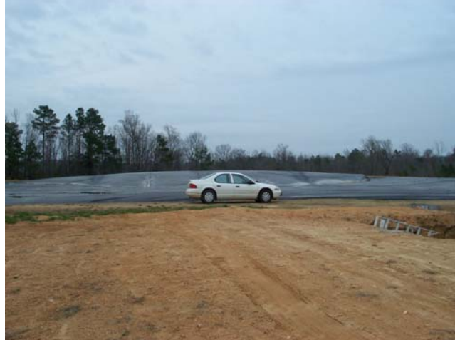
Figure 3. Enclosed anaerobic lagoon that produces biogas for energy. The cover swells due to the gas production inside.
