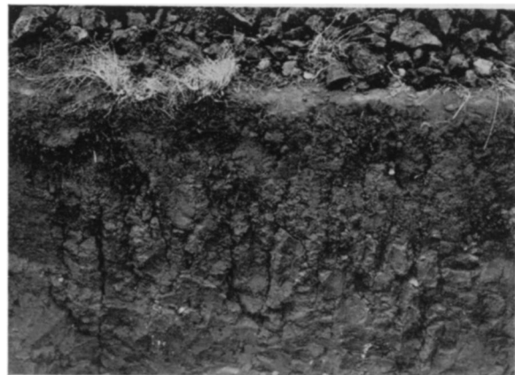
FIG. 48. Wall of trench where root systems were examined showing dried and cracked soil to a depth of about 4 feet. Pleasant Dale, Neb., July, 1940.
