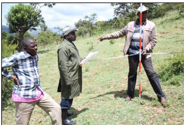
Laying out of plot
