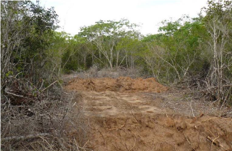
Figure 24. Prospecting outline 'sealed off' using bulldoz- ers and cut branches, Palma area.
