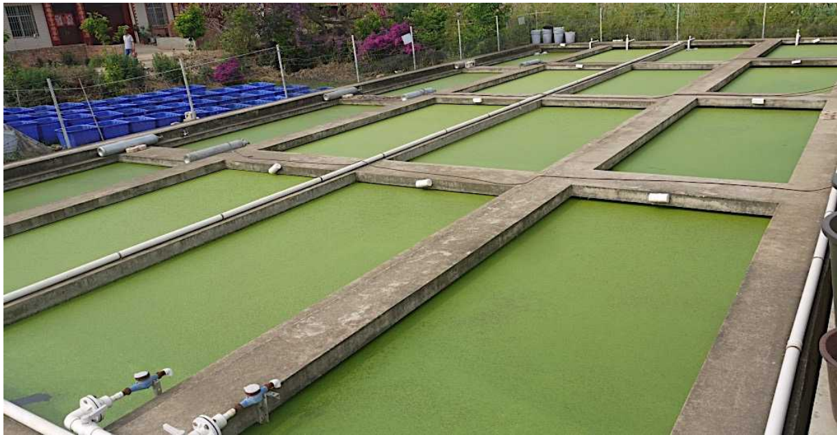
Figure 2: Duckweed wastewater treatment system in Yunnan
